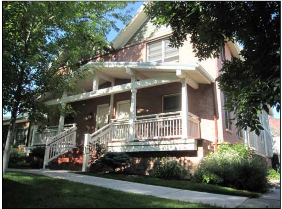
Infill projects such as this one in downtown Glenwood Springs, CO, can capture growing demand for centrally located housing in walkable neighborhoods.
